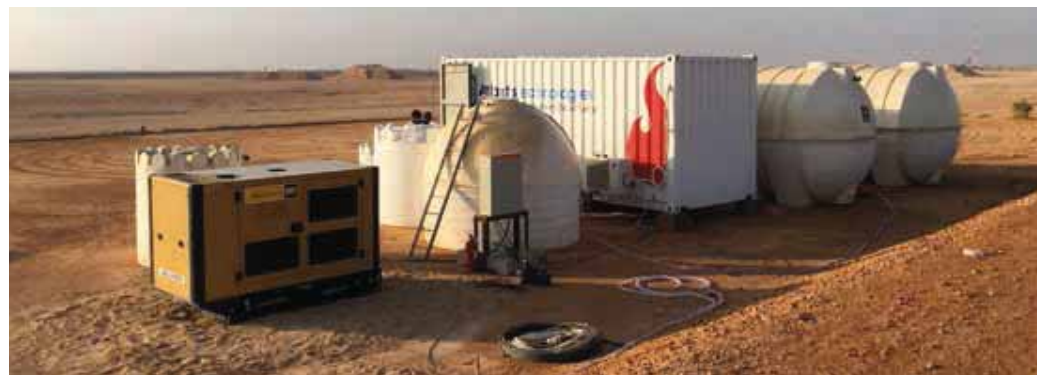
Containerized Atlantis RDI system with generator and water storage tanks at Bauer Nimr. Photo by Atlantis Technologies
